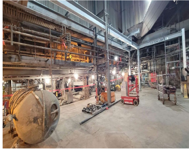
Unit 5 basement - March 2024
